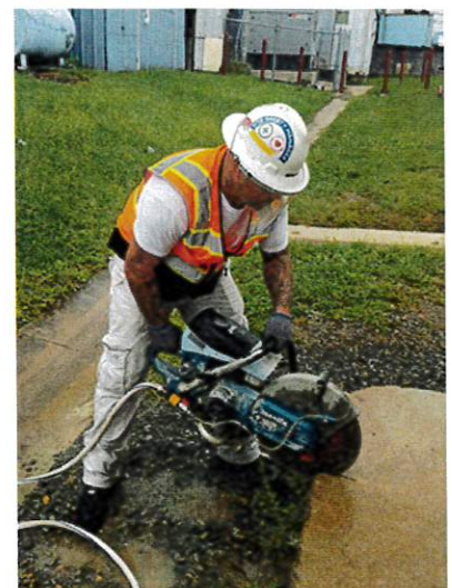
Applying water to a saw blade when cutting materials that contain crystalline silica — such as stone, rock, concrete,
